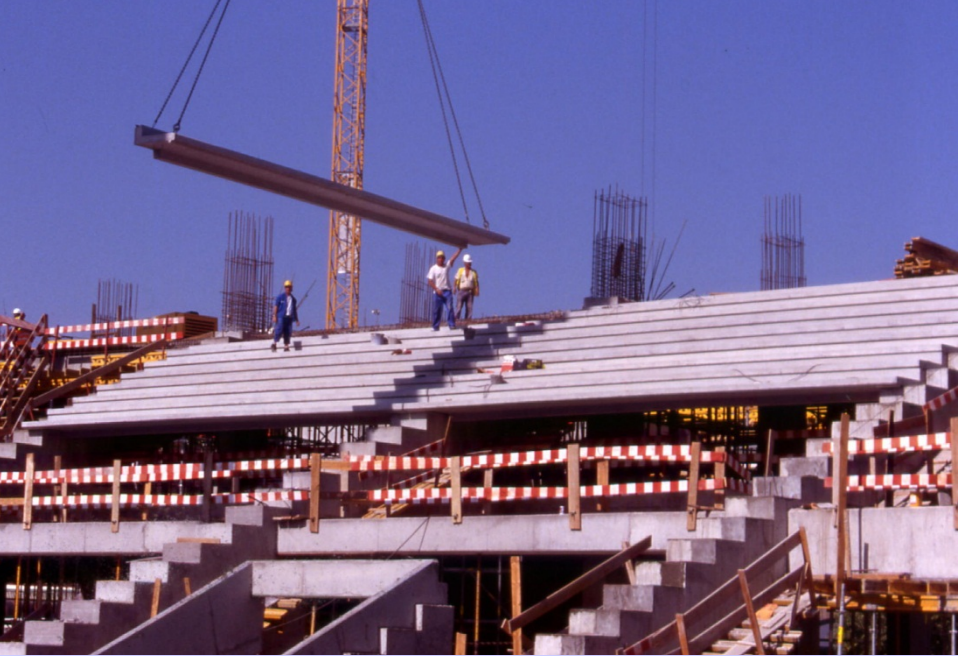
with c-i-s concrete
