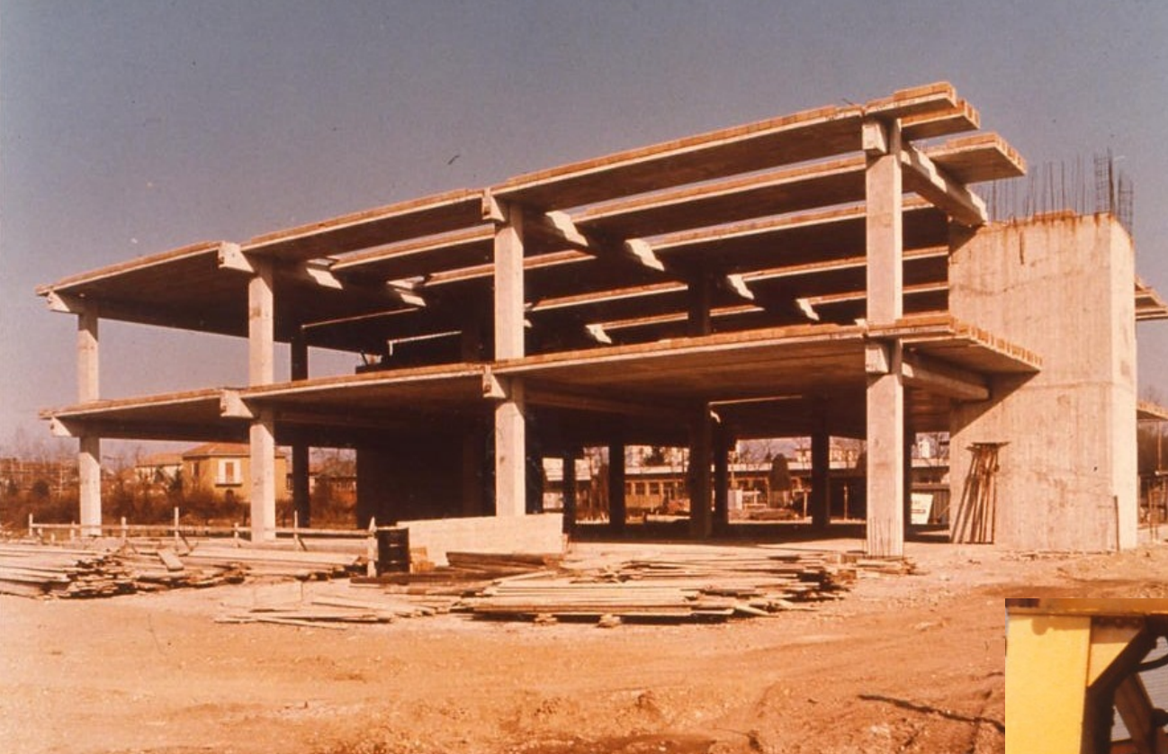
early 1950's precast prestressed floor patent
