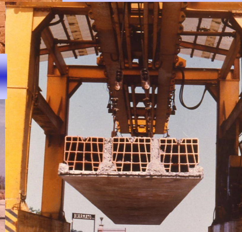
early 1950's precast prestressed floor patent
