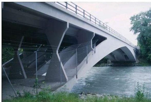
Vessy Bridge (Maillart, 1937)
