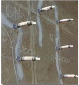
Crack injection (injecting resin)
