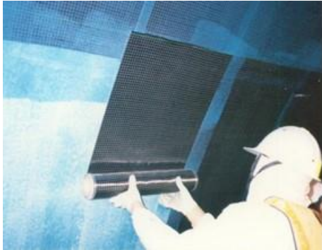
Prevention of concrete peel off (external bonding of FRP sheet)
