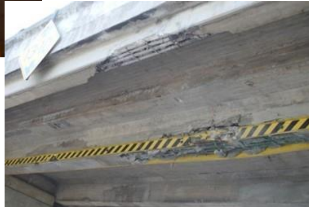
Snow overload, vehicle collision
