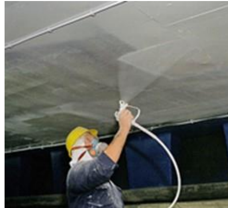
Surface protection (coating resin)
