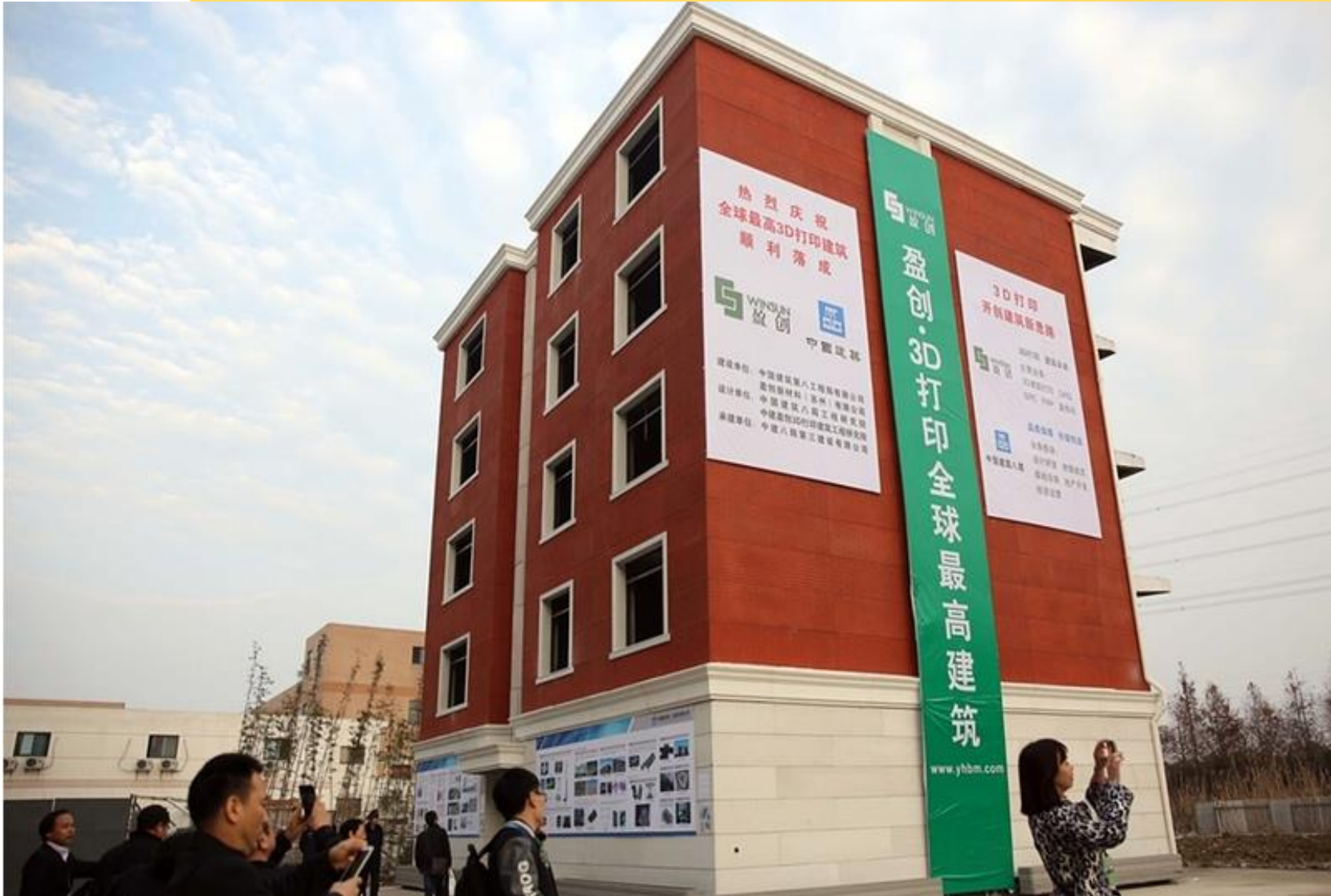
WinSun's 3D-printed building in Suzhou industrial park
