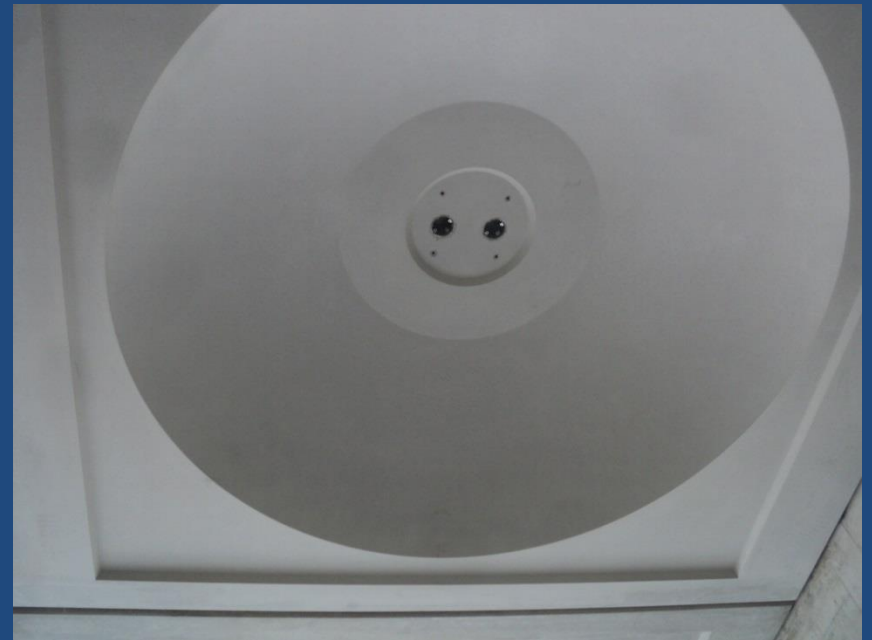
Precast Coffer Viewed from Below.
