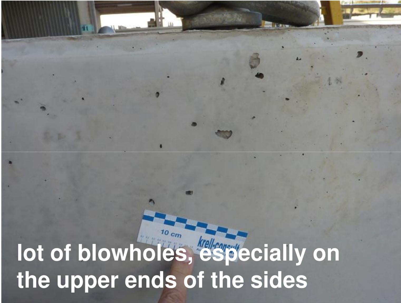
lot of blowholes, especially on the upper ends of the sides
