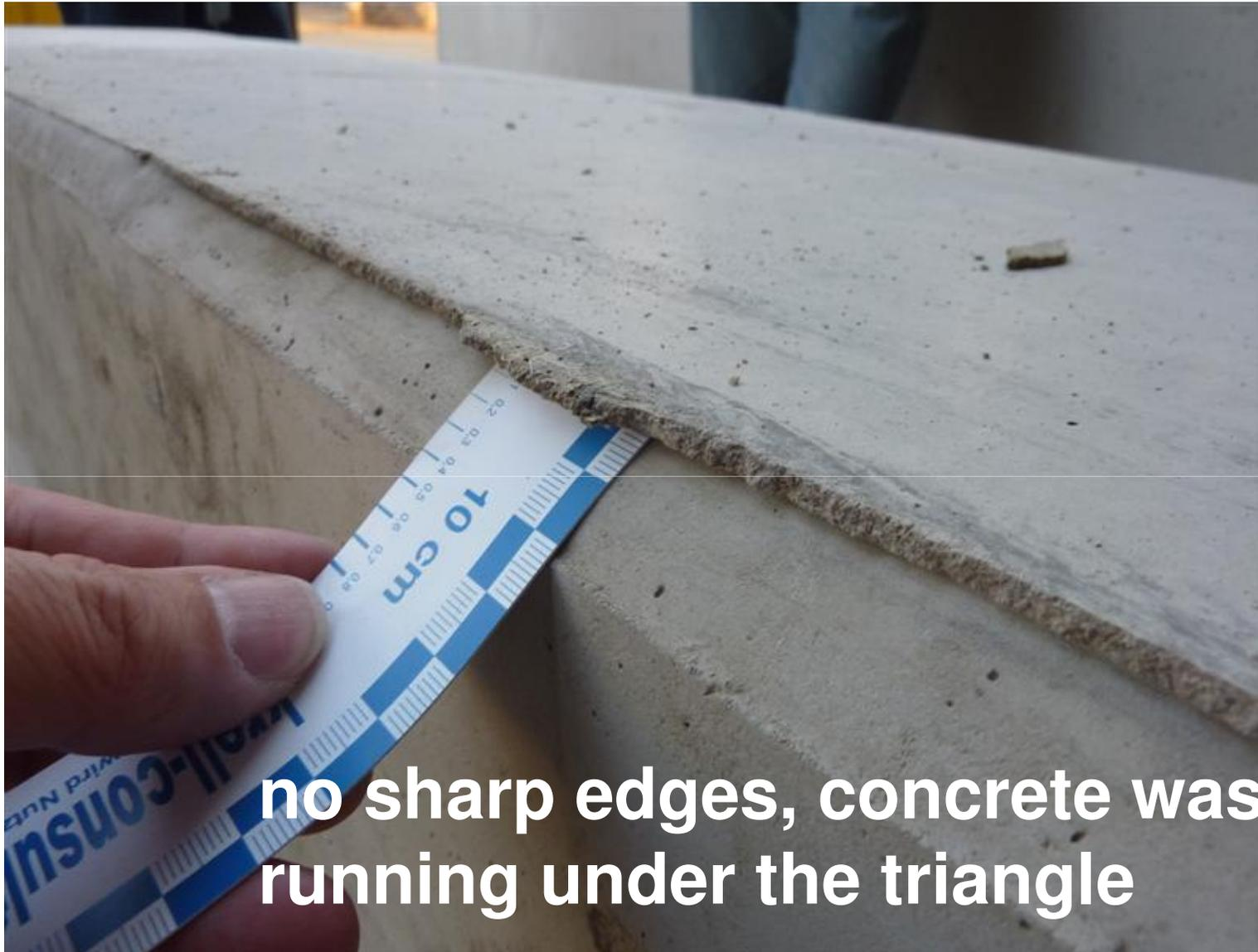
no sharp edges, concrete was running under the triangle
