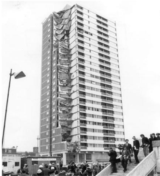
Fig. 1: Progressive collapse of part of 26 storey apartment building “Ronan Point” (1968)
